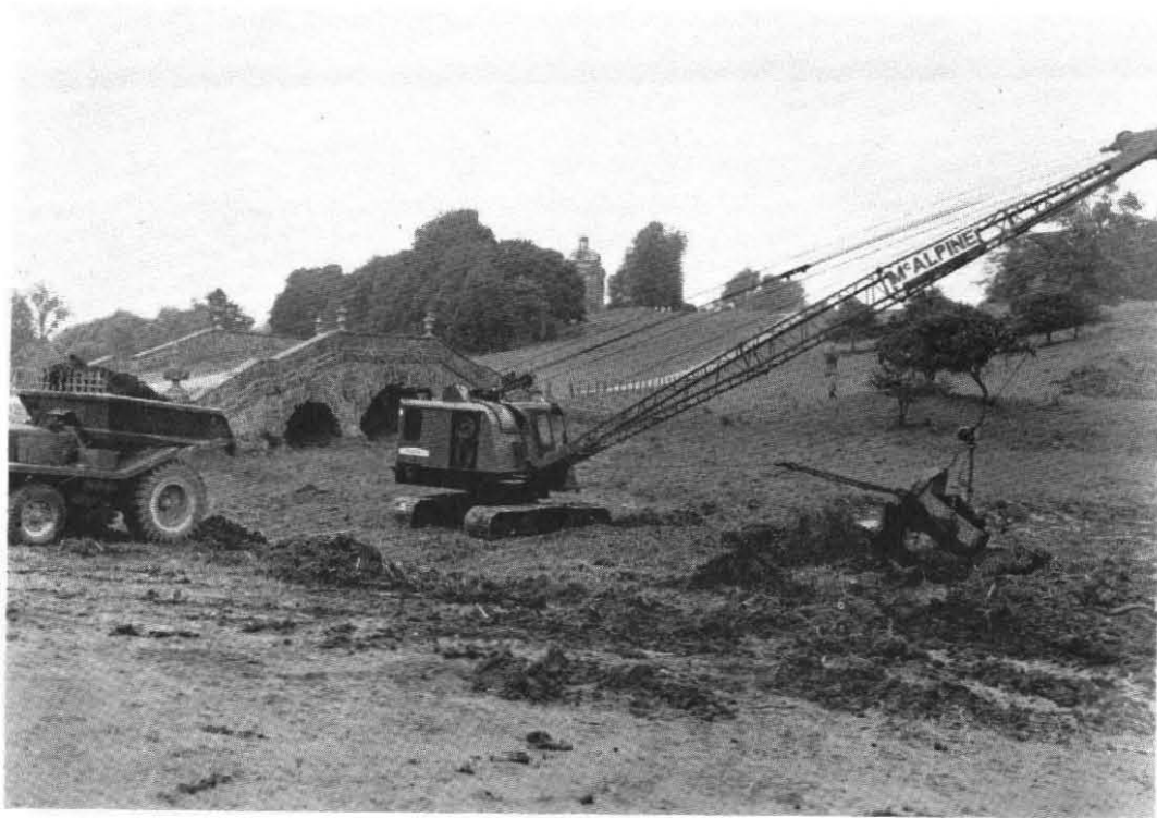
EXCAVATING THE SILT
