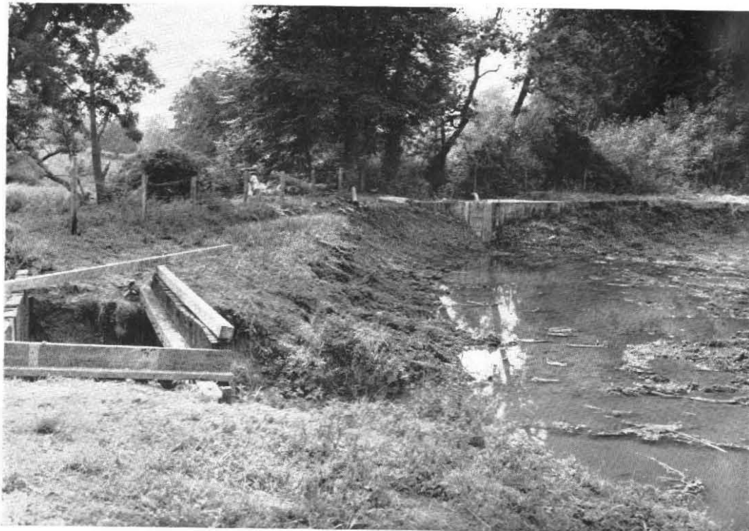
THE BREACH IN THE BANK AND THE NEW DAM
